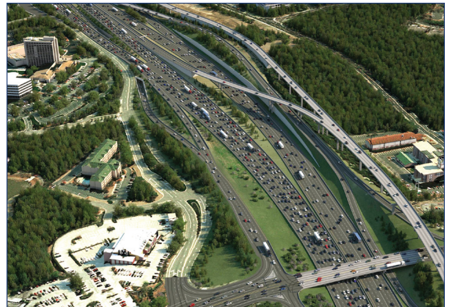
Artist rendering of the Managed Lane System Flyover at Windy Hill Road
